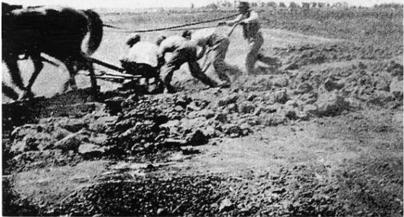
I-H TENNIS COURT CONSTRUCTION
