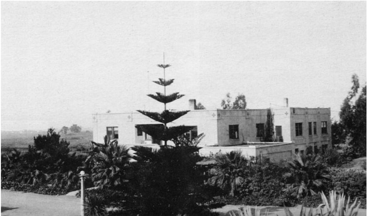
III - K Administration Building with Annex (Note Star Pine)
