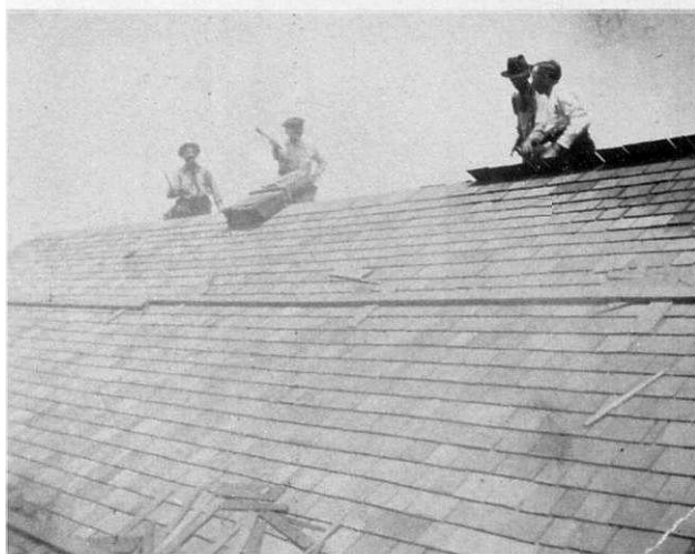
II-D Max Heindel and First Water System Crew Shingling Roof
